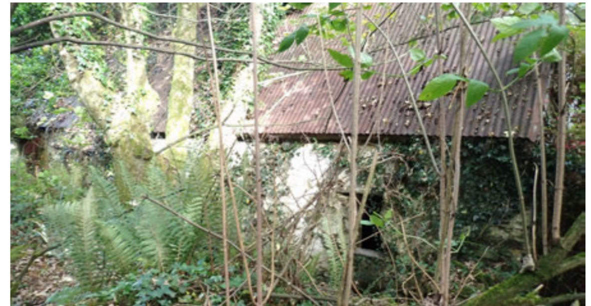
Photo 9.3.22 View of the overgrown old farmstead located in the wooded area,
