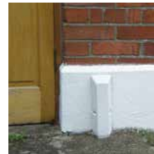
Service riser cover
